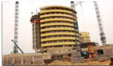
Skyline of PTDF Head Office Building under construction in Abuja
