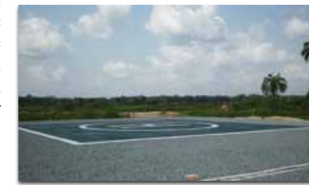
Completed Helipad of Federal Polytechnic, Ekowe
