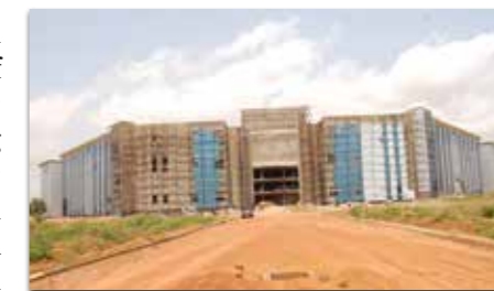
Int'l Conference Centre under construction
