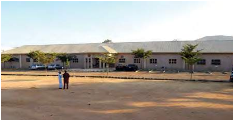
Front view of the fully equipped Mechanical Engineering Department constructed by PTDF at the Abubakar Tafawa Balewa University (ATBU), Bauchi
