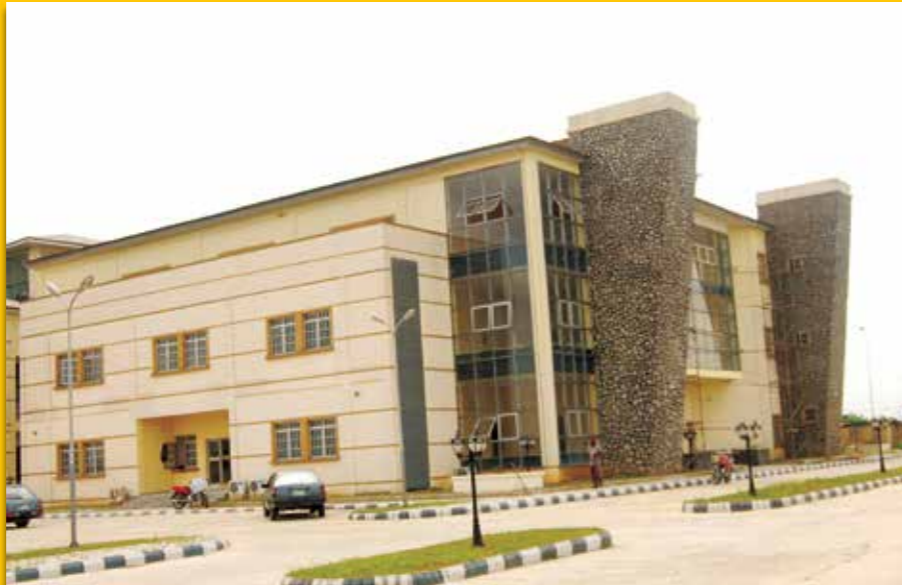
The Training Centre at the Petroleum Training Institute, Effurun, Delta State
