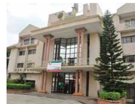
PTDF old office building in Port Harcourt Crescent, Area 11, Garki, Abuja
